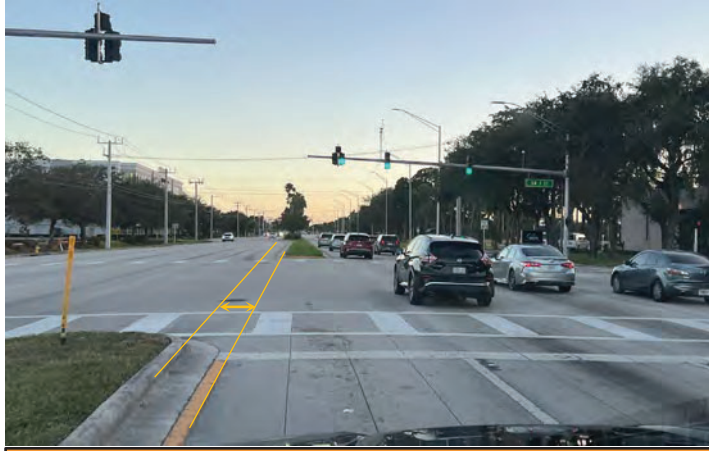
Existing offset of the left-turn lanes. Looking south.
