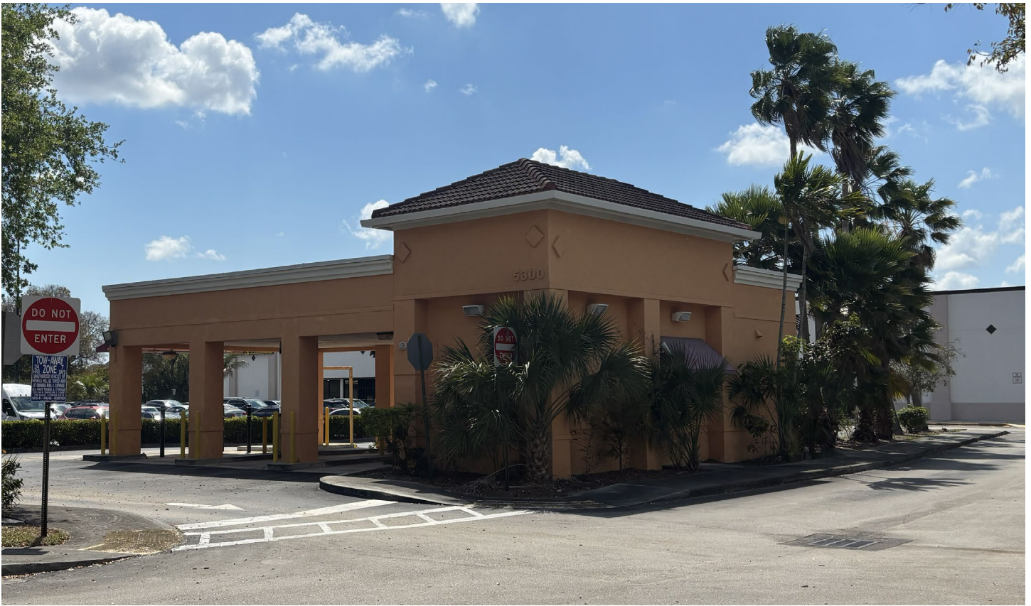
[Subject Property Current Condition – North and West Façade, March 26, 2026]
