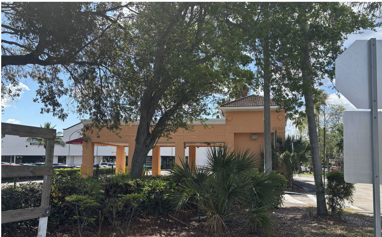
[Subject Property Current Condition – North Facade, March 26, 2026]
