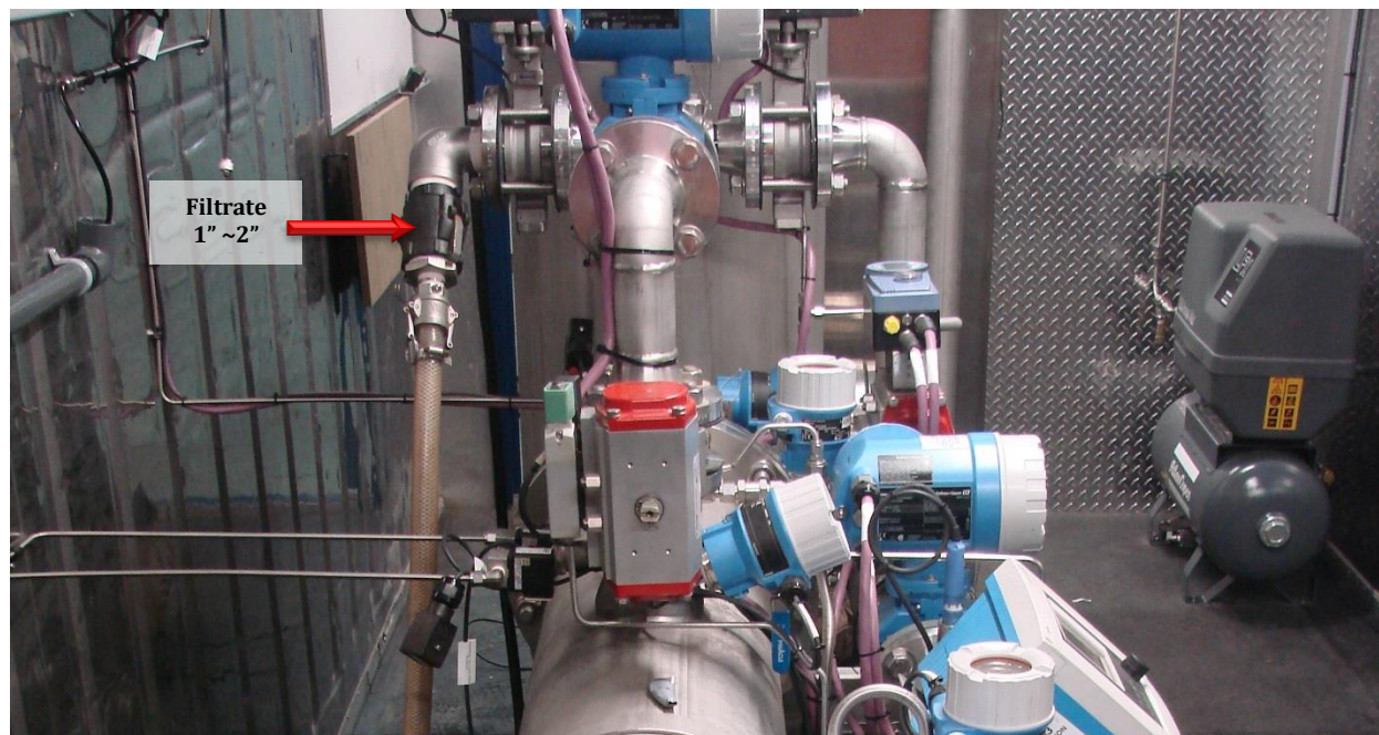
Figure: Cuf Filtrate Connection
