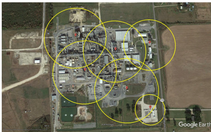
Chemical Plant - Example Only
