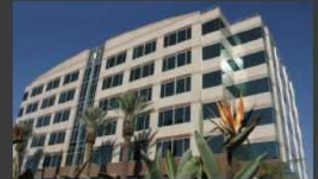
L.A. County Building - Phase 2 Department of Children's Services El Monte, California
