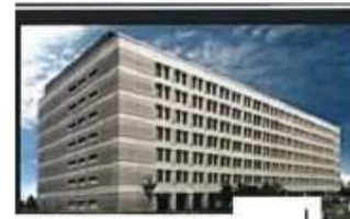
Department of Homeland Security L.A. Headquarters Building Norwalk, California
