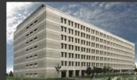
Department of Homeland Security L.A. Headquarters Building Norwalk, California
