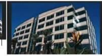
L.A. County Building Phase 2 Department of Children's Services El Monte, California
