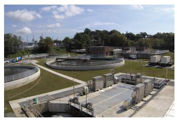
An AECOM JV was awarded a design-build-operations contract to upgrade the City of Newport's Water Pollution Control Plant (WPCP). This project involved upgrading the WPCP to a 30 mgd maximum daily flow limit and also included new rotary drum thickening and dewatering systems. Key scope items for the upgrade included:
