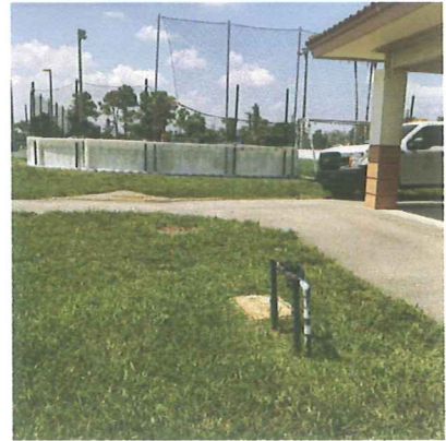
Existing Water Service
