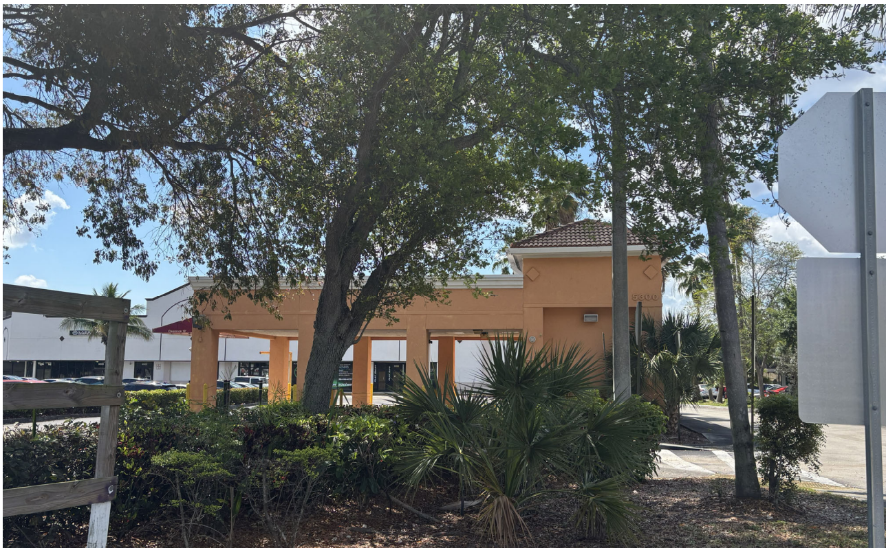
[Subject Property Current Condition – North Facade, March 26, 2026]
