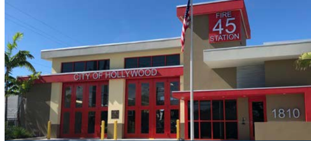
Hollywood Fire Station 45
