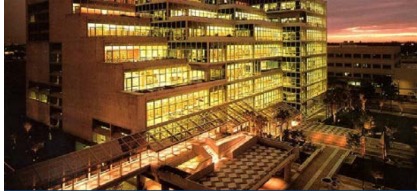
Broward Main Library Wind Mitigation & Hurricane Hardening
