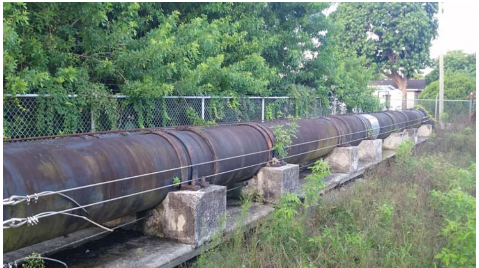
Existing pipelines are supported by concrete cradles that rest on a pile cap.
