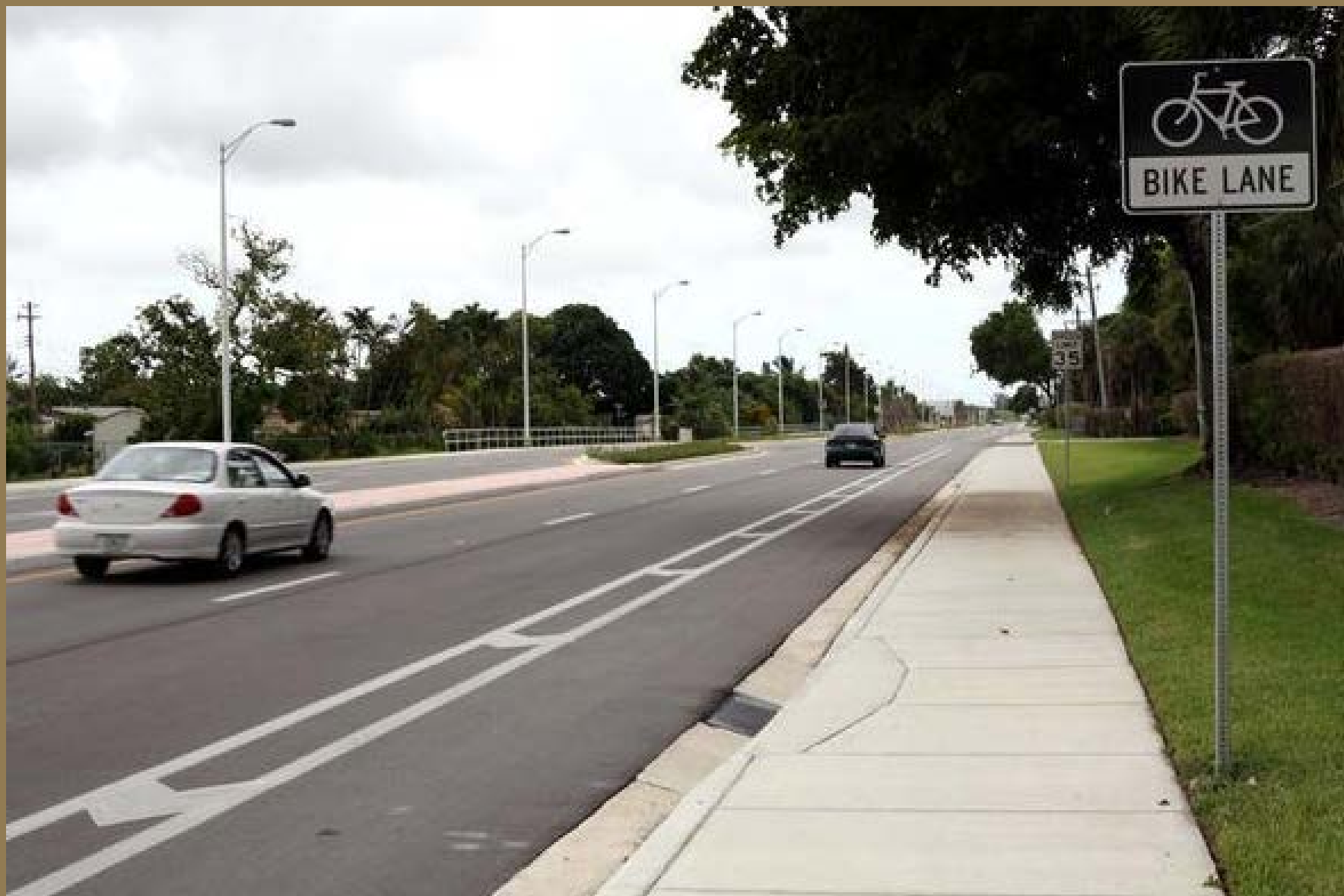
NW 62 Ave / NW 31 St – Buffered Bike Lane
