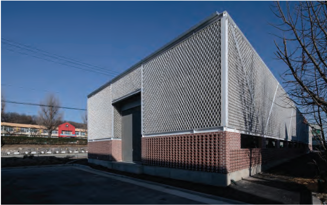
GOOD EXAMPLE: Warehouses can be architecturally innovative and elegant. In this well-proportioned example, a brick base with a textured pattern supports a steel frame infilled with fragments of recycled PVC pipes.
